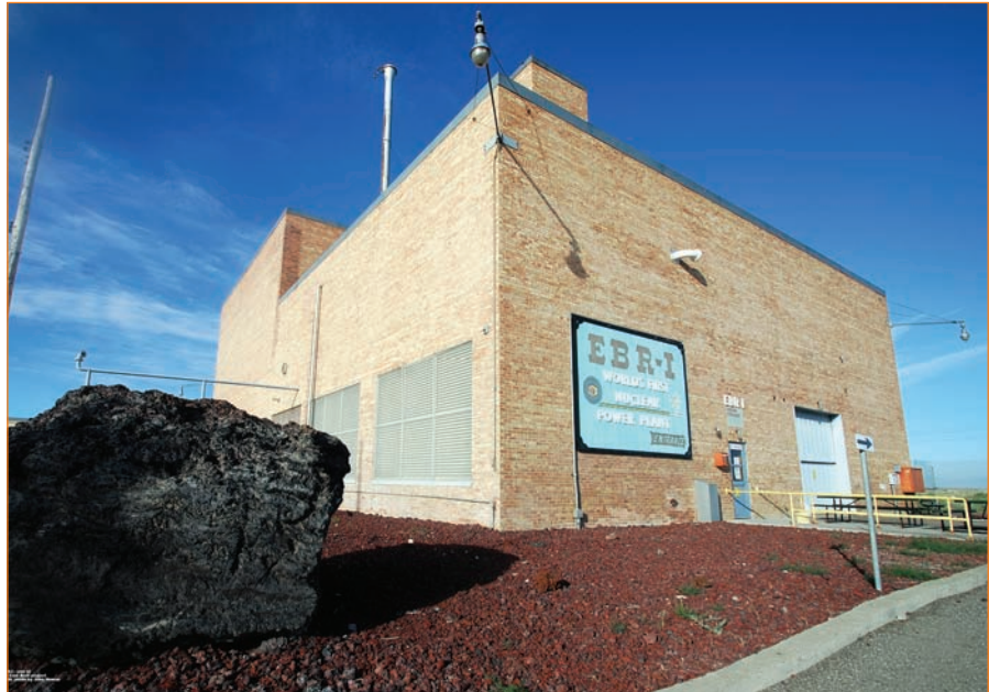
Photo courtesy of Idaho National Laboratory
