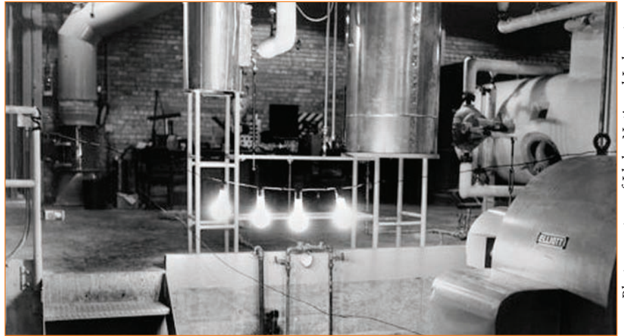
On December 20, 1951, four light bulbs were strung from the generator (right bottom corner) and they were lit. It was the first time in the world a reactor made that much electricity.
