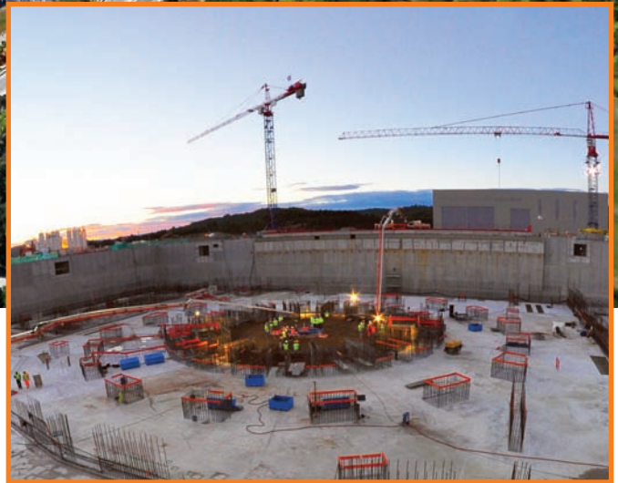
The final pour of the Tokamak Complex floor.
