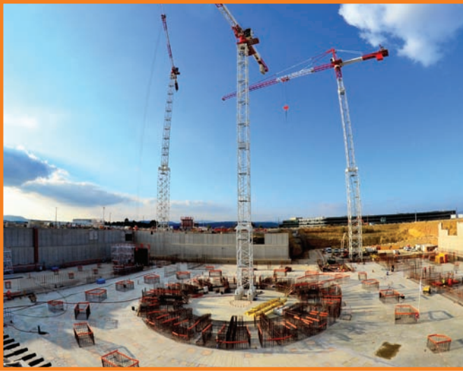
Tokamak Complex under construction.
