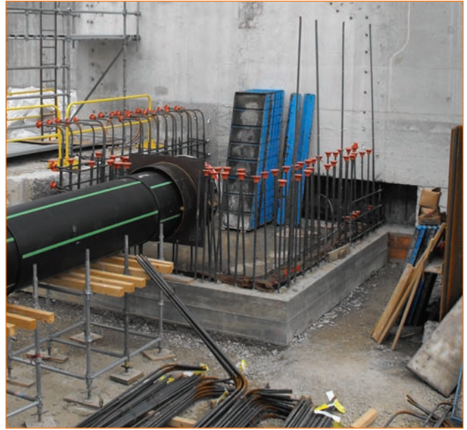
HDPE pipe installation through sleeve into heat exchanger building.
